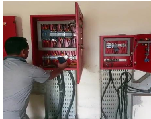
Gambar 3. Komponen panel Jockey Pump
