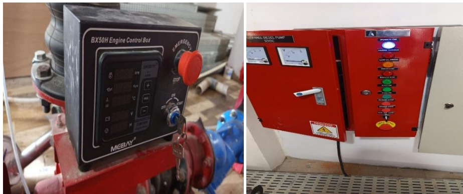
Gambar 5. 1 Panel control standing diesel. 2 panel kontrol utama diesel
